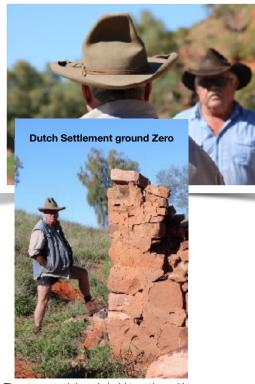
The stone work here is held together with mud mortar, no cement, which is not surprising.
