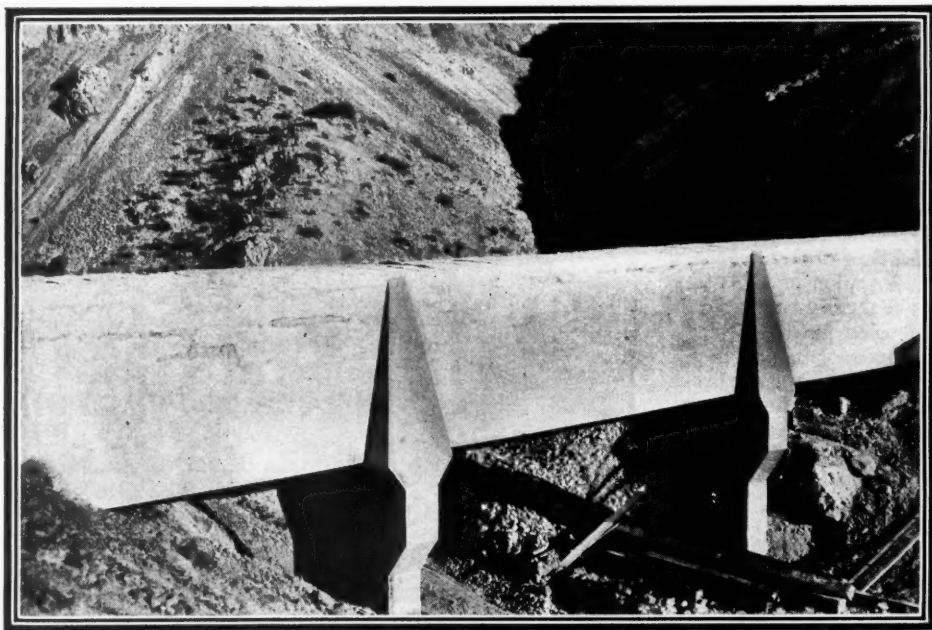
ONE OF THE CONCRETE FLUMES IN THE JAWBONE DIVISION OF THE AQUEDUCT
