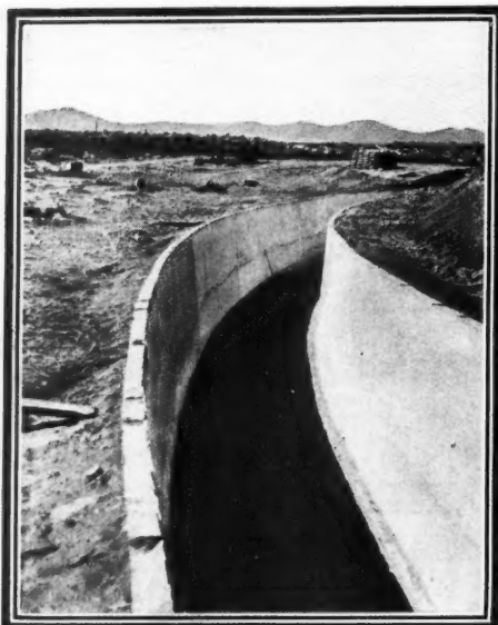
A VIEW OF THE CONDUIT IN THE DESERT, LINED AND READY FOR COVER
